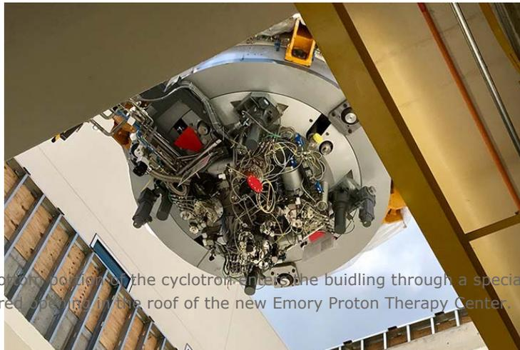
The bottom portion of the cyclotron enters the building through a specially prepared opening in the roof of the new Emory Proton Therapy Center.
